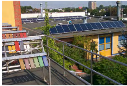
Photo-voltaic and solar heat installations
